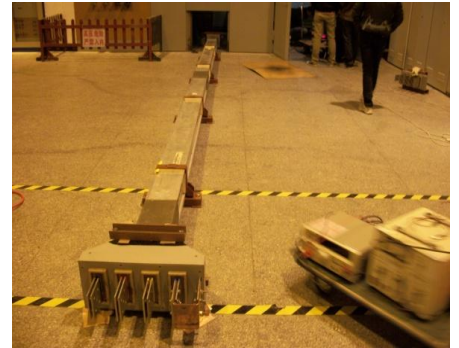
Clause 8.2.4.2 : Verification of effectiveness of the Protective Circuit (Icw) – Feeder Elements without Tap-off Unit
