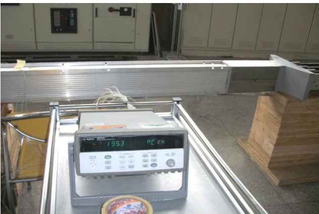
Thermal With-Standability Test Setup
