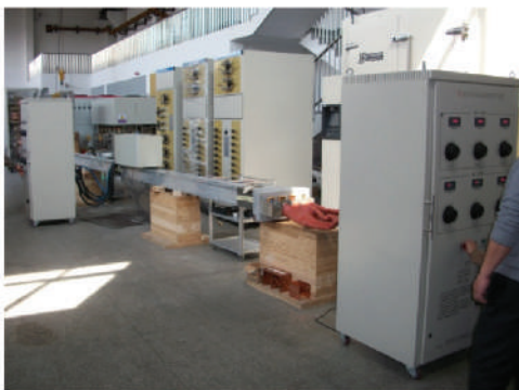
Clause 8.2.6 : Verification of Mechanical Operation
